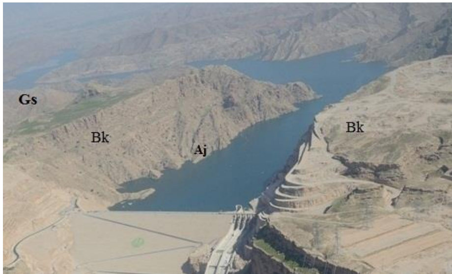
Fig. 2 – An upstream (eastward) view of the Upper Gotvand dam reservoir and the outcropped formations; Bakhtyari (Bk) Conglomerates, Agha-Jari (Aj) Sandstones, Gachsaran (Gs) Evaporates
